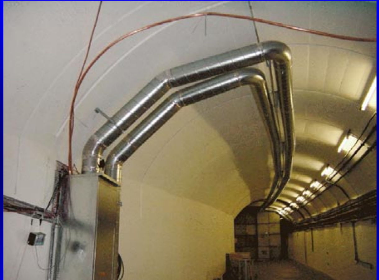
Cupboard for the Inflammable gases
